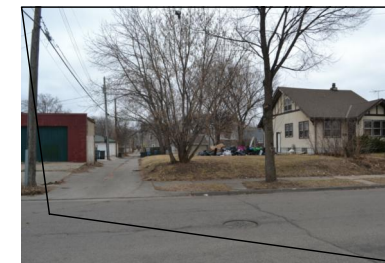
FRONT OF 1818 SHERIDAN AVENUE NORTH CITY OF MINNEAPOLIS, HENNEPIN COUNTY, MN
